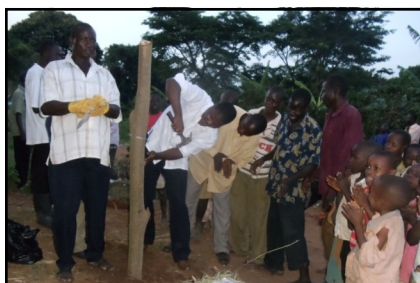
Fencing of the property begins!
