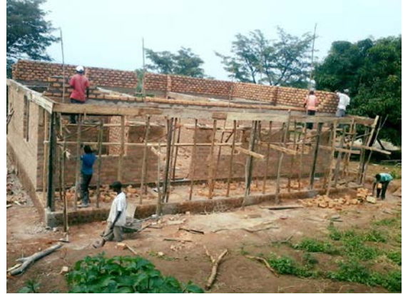
The foundation is laid and the walls are going up!
